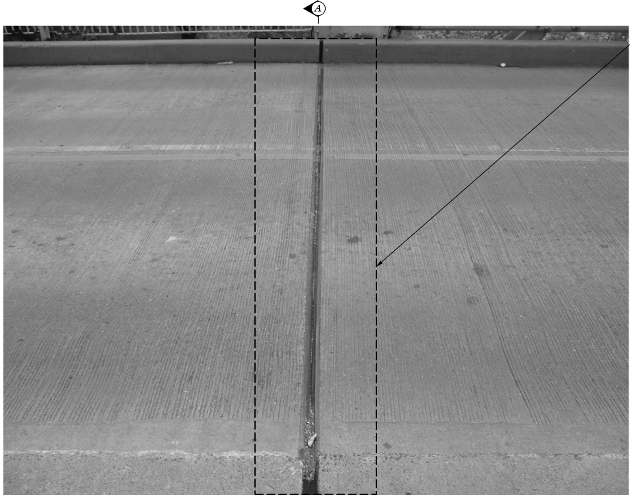
REPAIR 7 JOINT SEAL REPLACEMENT
