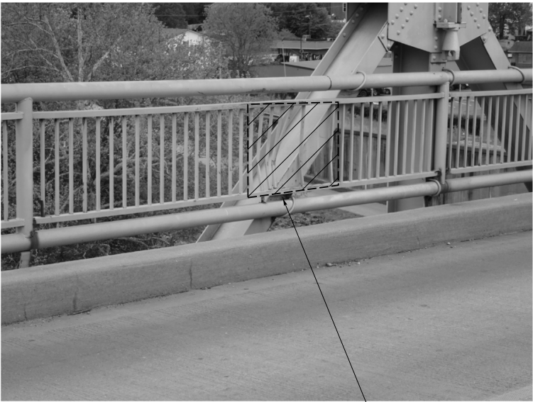
Replace Deteriorated Rail Elements
