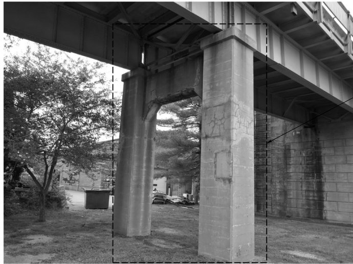
Concrete Patching and Coating of Substructure Units
