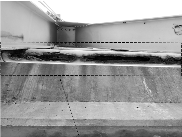
Replace Deteriorated Rail Elements
