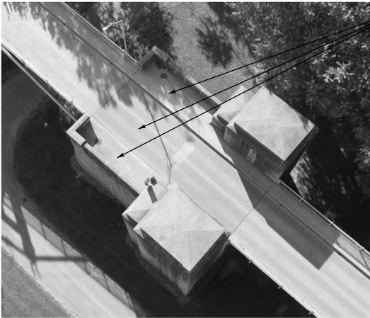
Epoxy Overlay top of slab and sidewalk
